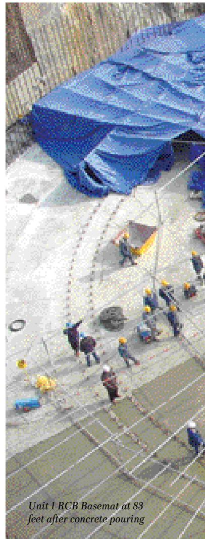
Unit 1 RCB Basemat at 83 feet after concrete pouring
