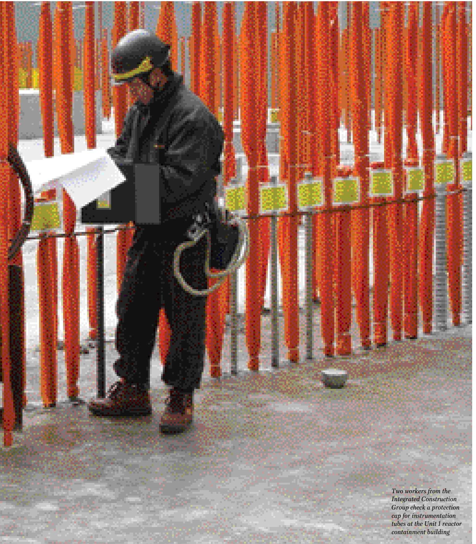
*Two workers from the Integrated Construction Group check a protection cap for instrumentation tubes at the Unit 1 reactor containment building*
